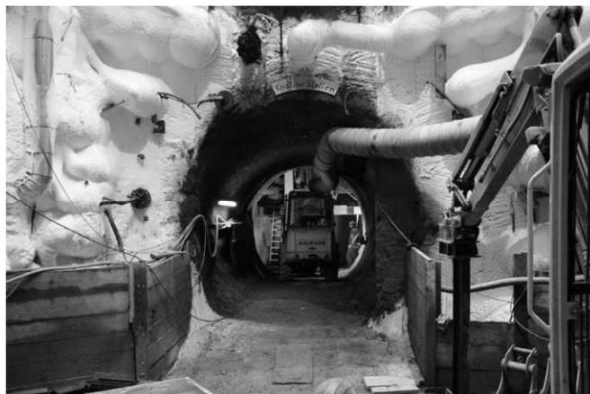
Figure 10 Tunnel drift protected by ground freezing.
