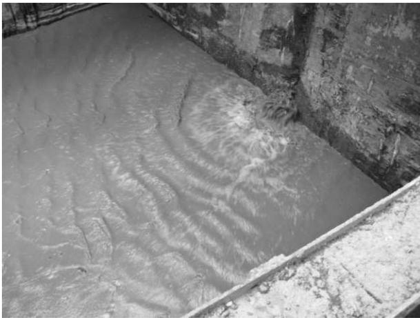
Figure 13 – Water and sand entering the excavation
