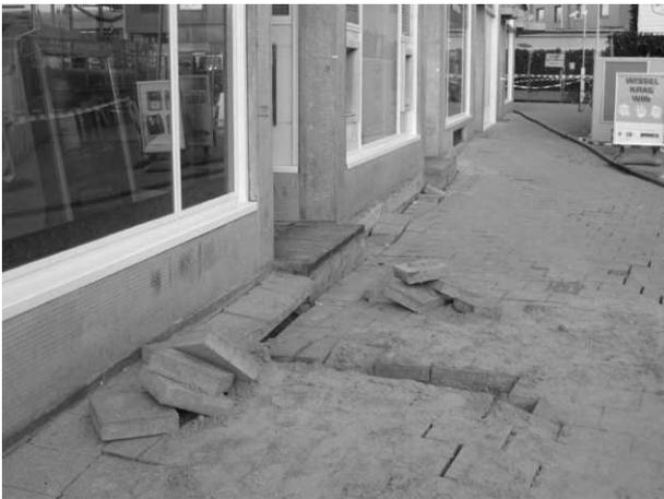
Figure 17 – Settlement caused by wash-out of deep sand layer.
