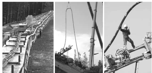
Fig.10. Assembly and installation of anchors
