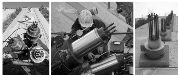
Fig. 9. Stressing the Anchors
