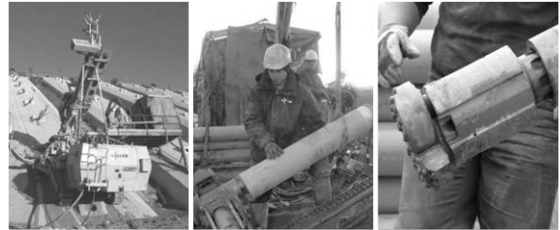
Fig. 8. Drilling situation and used tools
