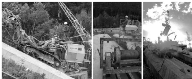
Fig. 11. Steps to move the rig to the drilling position
