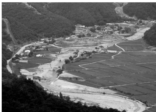
Figure 3. Overview of debris flow affecting a rural community.
