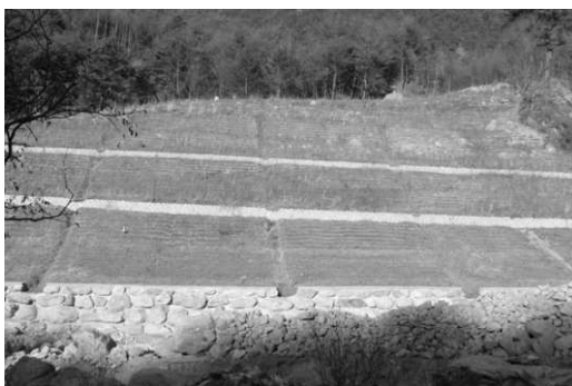
c) A slope protected by the seed spray method
