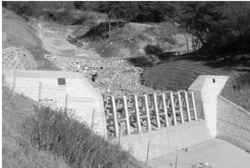
a) A slit-type debris barrier
