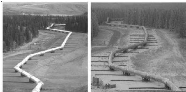
Figure 1. Pipe Location: Pre-Earthquake (Left) Post-Earthquake (Right), (William et al, 2003)
