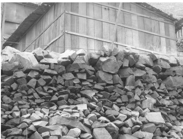
Figure 7. Typical Foundations on “Pircas”
