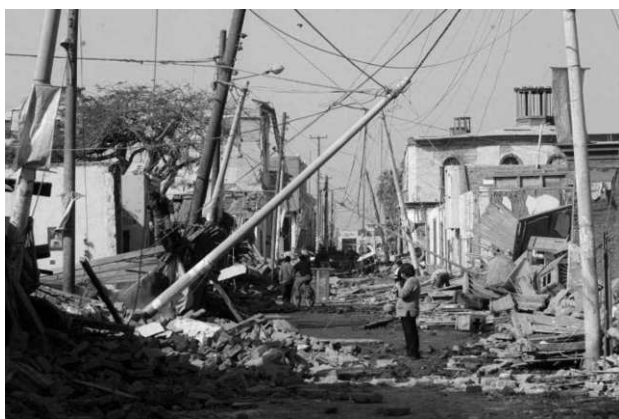
Figure 2. Earthquake Damages Pisco, Peru, August 2007
