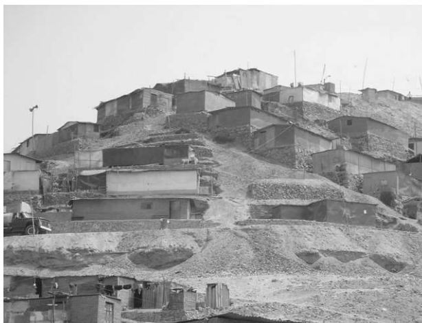
Figure 4. Placement of households with unstable foundations
