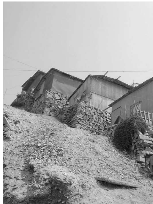
Figure 8. Staggered Terraces built with “Pircas”
