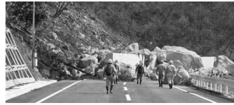
a) Case History of Rockfall Failure in Japan
