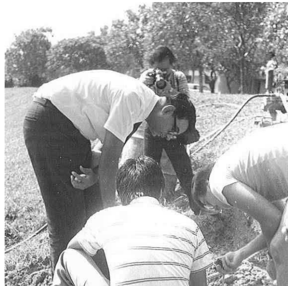
Author with NTI students installing an inclinometer.
