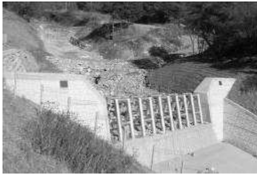
a) A slit-type debris barrier
