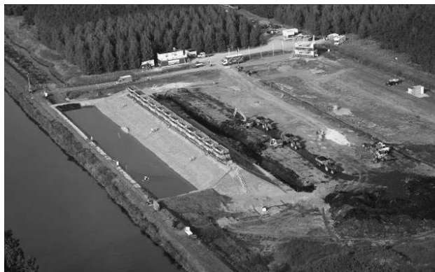
Fig 3: IJkdijk stability test
