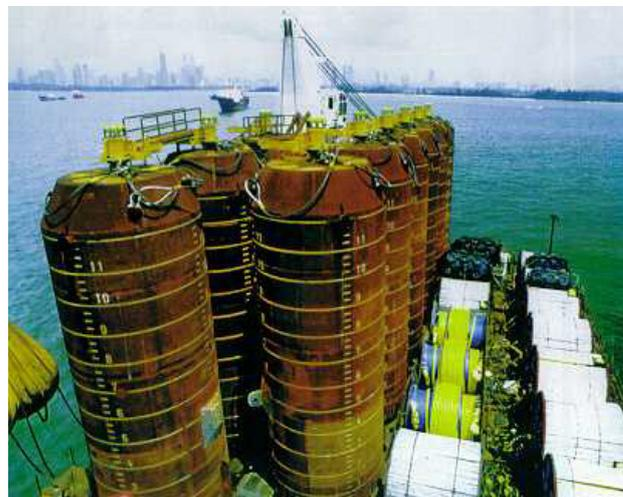
Figure 6.3 Suction caissons for the Laminaria field in the Timor Sea.
