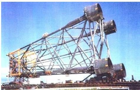
Figure 4.9 Draupner E jacket with steel bucket foundations (© NGI)
