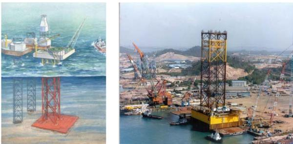
Figure 4.7 Yolla A Hybrid gravity base structure, Bass Strait, Australia (Watson & Humpheson, 2005)
