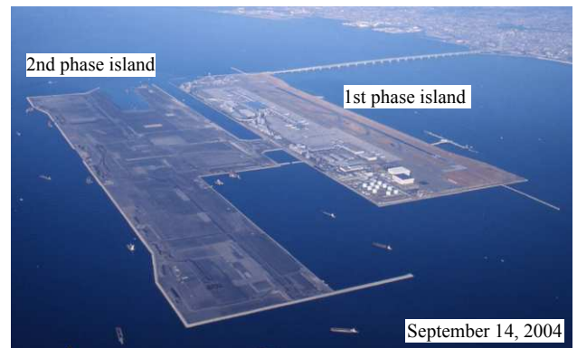
Figure 4. Overview of the first and second airport island of KIA
