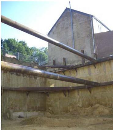
Fig 9: CSM wall (Holland) after excavation
