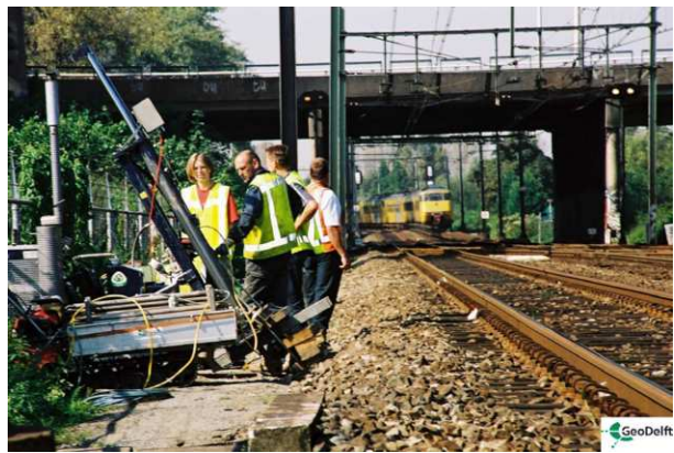
Figure 3: Execution of an inclined CPT.
