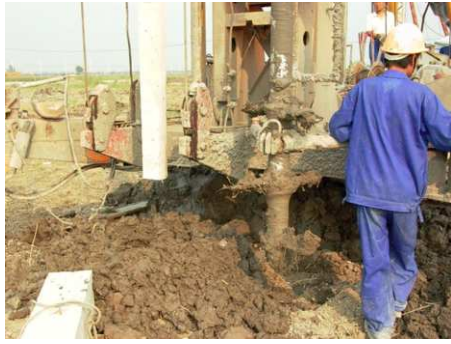
Figure 7. Mini pile driving after DMM column installation
