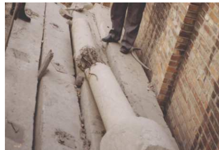
Figure 10. Crush of mini pile exhumed after loading test
