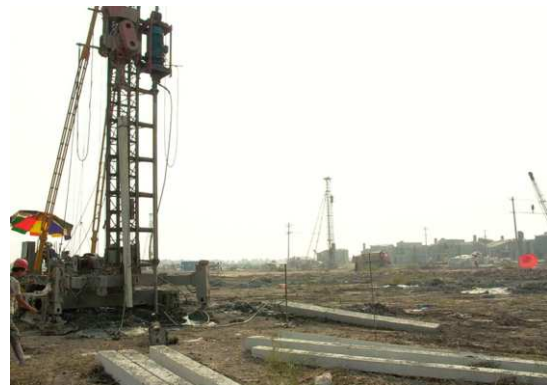
Figure.12 Mini reinforced concrete piles used in Dongli Lake
