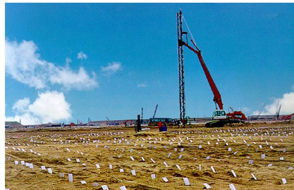
Fig. 3 Installation of plastic board drain
