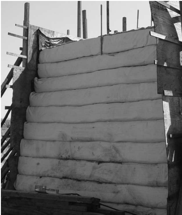
Figure 1 – Geotextile reinforced soil retaining wall
