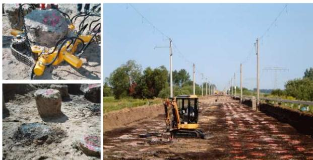
Fig. 10. Cutting the pile heads (left) and removed embankment (right)
