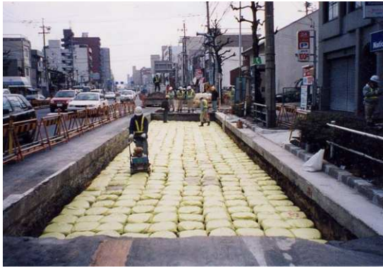
Figure 6. Reinforcement for an asphalt-paved truck road with soilbags.
