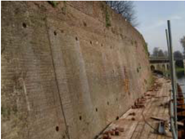
Figure 7.1 Removal of the brickwork for the nailing
