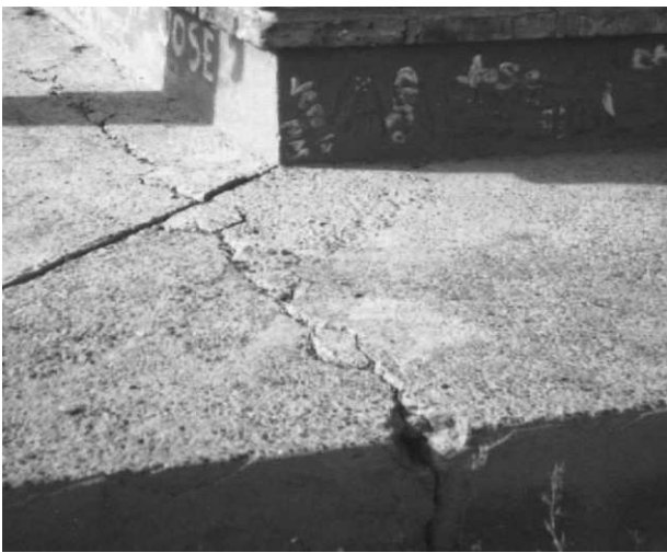
Figure 2. Cracked footpaths.
