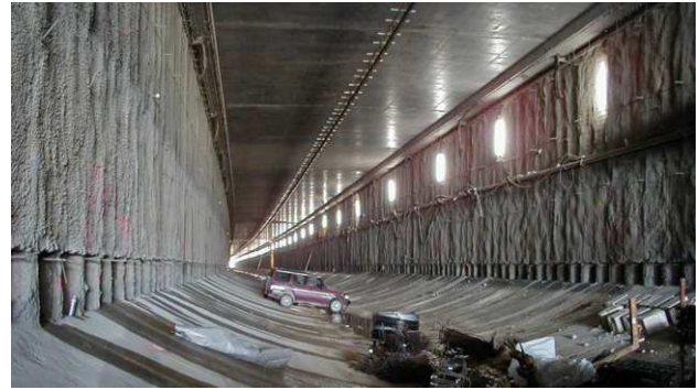
Figure 9. Construction of the invert (temporary)
