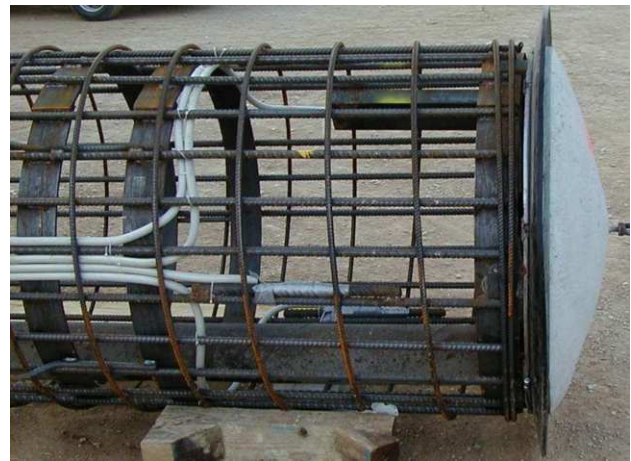
Figure 4. measuring systems for the pile loading test
