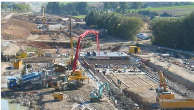
Figure 7. Construction of the tunnel roof (top cover)
