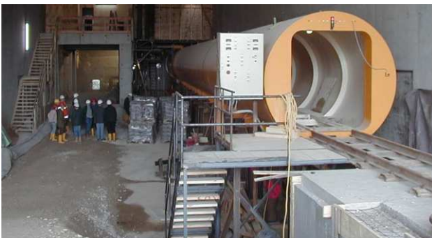
Figure 8. Compressed air driving – air lock
