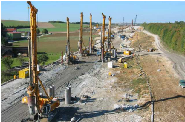
Figure 6. Construction of the watertight bored pile walls
