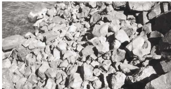
Figure 2 – Upstream protection rockfill of Marimbondo dam.
