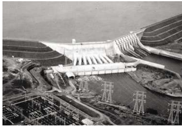
Figure 1 – Aerial view of Marimbondo dam and power plant.
