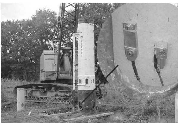
Fig 1: Hammer, pile and transducers details of a Dynamic Load Test
