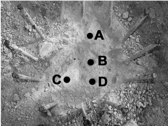
Figure 3. Outline of the positions A-B-C-D at a pile head.
