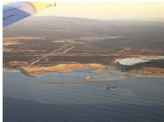
Figure 5: Flooded harbour in August 2004.
