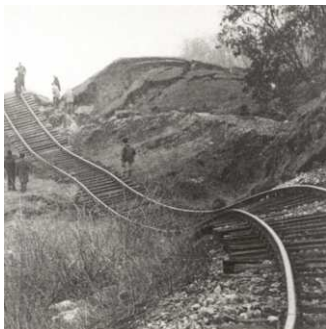
Figure 5. Railway failure in the bulging zone
