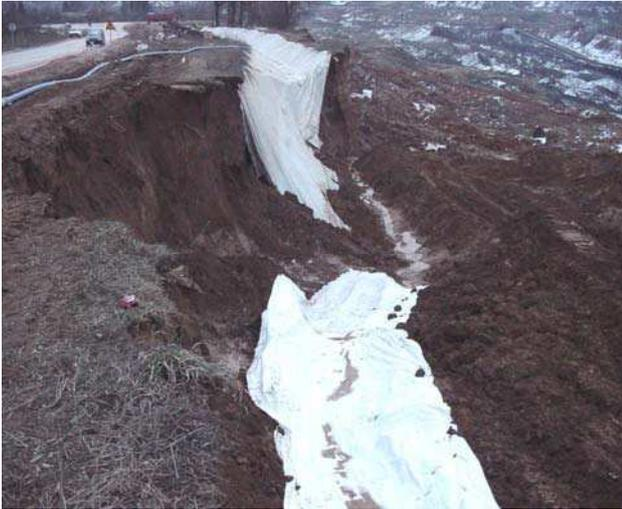
Figure 2. Land sliding about profile IV - condition on the 11 February 2003
