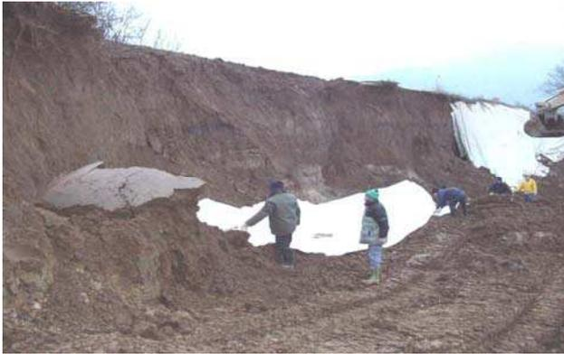
Figure 5. Construction of the first layer of Comtrac on the upper retaining wall of system reinforced earth
