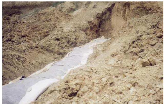
Figure 4. Designed and constructed drainage prism
