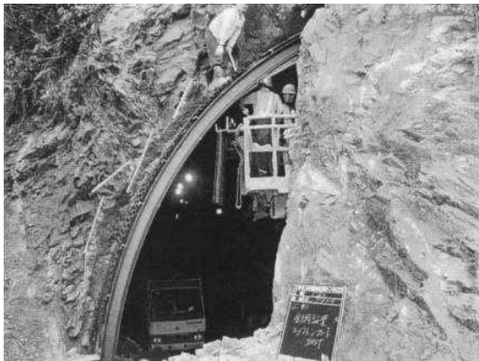
Photo 1 Situation immediately after the entrance was cut through
