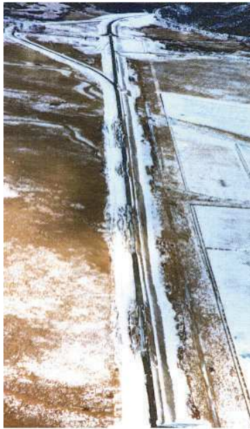
Figure 10. Aerial photograph of Kushiro River dike showing failed sections at periodic intervals (Kano et al.)
