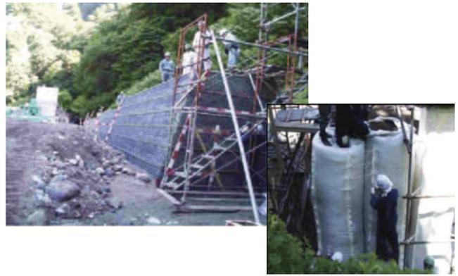
Photo 17. RE combined with impact absorber.
