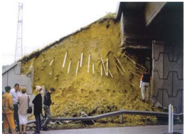
Photo 9. Case study for failure of reinforced soil wall (from presentation by Prof. Sharle)
