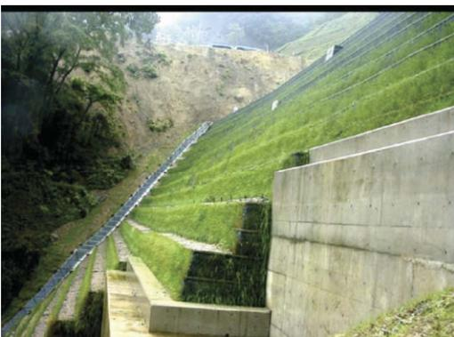
Photo 16. RE combined with PLPS and drainage.
