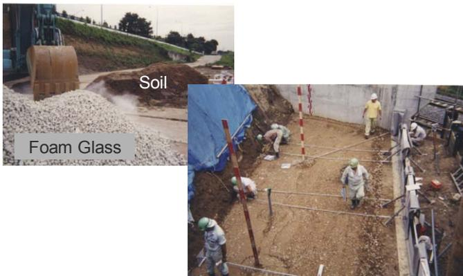
Photo 14. RSW combined with foam glass mixing.
