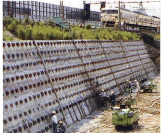
Photo 18. Nailing combined with deep mixing.
