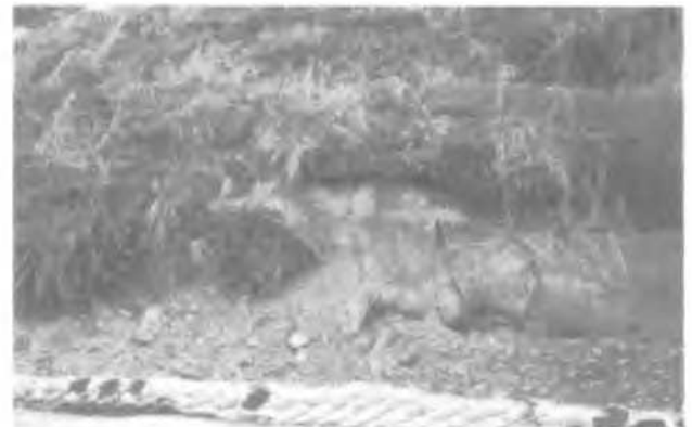
Figure 7. Separation between the adjacent geogrid layers.
