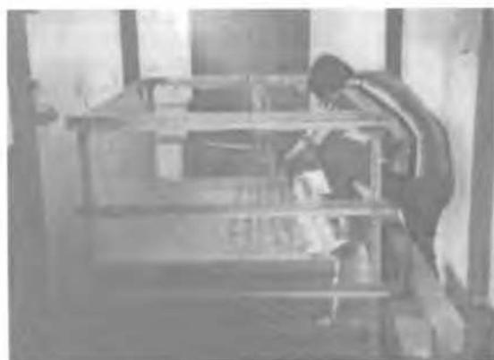
**Figure 9 – Construction of Bamboo Reinforced Walls**
