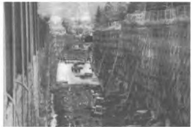
Figure 4. Excavation pit with soldier piles (left) and anchor wall (right)
