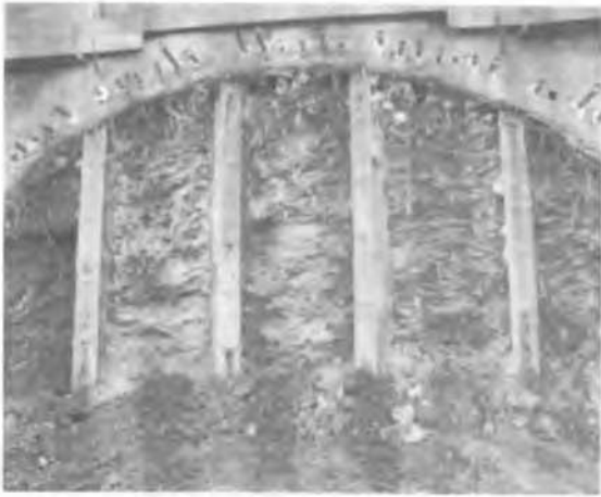
Figure 9. Start of top heading under the protection of umbrella
