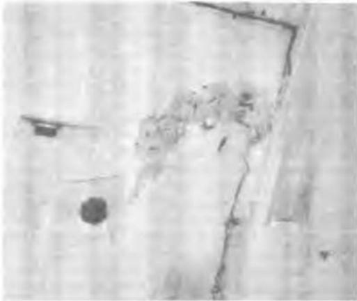
Figure 15. Damage to the tunnel lining; i.e. damage near the dowel and notch system
