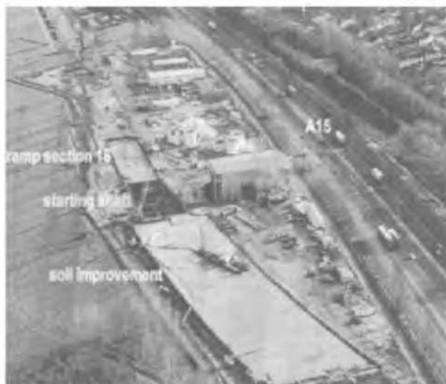
Figure 1. Construction of the starting shaft.
