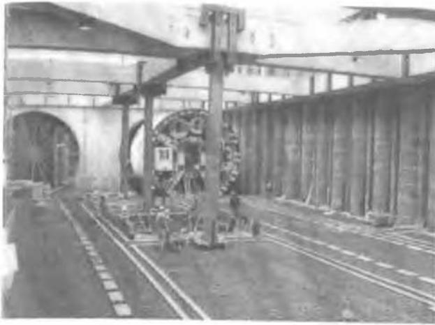
Figure 7. The starting shaft with part of the TBM assembled.
