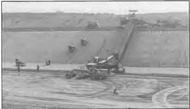
Figure - 5 Compaction of filter on power channel slope by rollers working in yo-yo system
