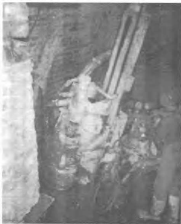
Fig. 10 Soilcrete works in a limited space in cellar
