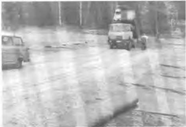
Figure 2: Dumping of the crushed gravel on the geotextile.
