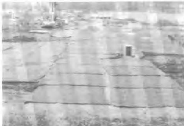
Figure 3: Geotextile sheets folded over the first embankment layer.
