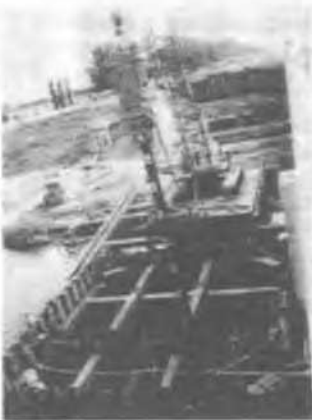
Fig. 3 The installation of H-pile in cofferdam
