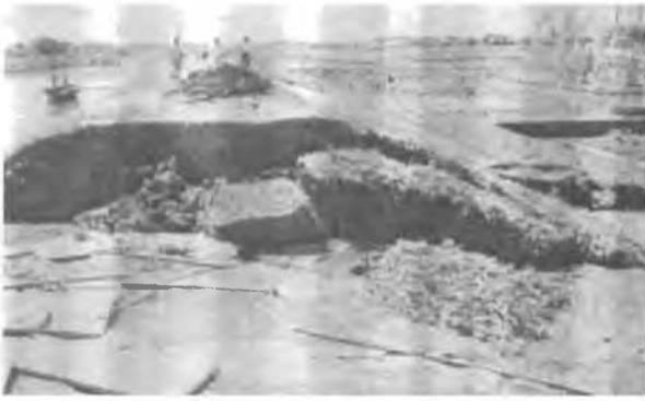
Figure 2. Piping failure of a clay dike (Nagoya, Japan)
