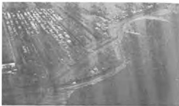
Figure 10. Test site at Bergambacht
