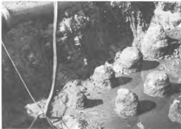
Figure 5. Excavation works in progress.
