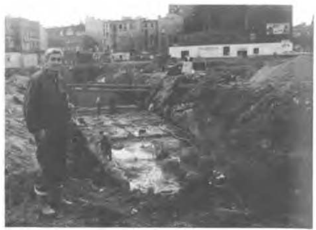
Figure 6. Building pit after excavation to the final depth.
