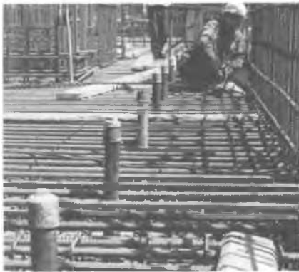
Photo 1 The situation of installation of grout tubes
