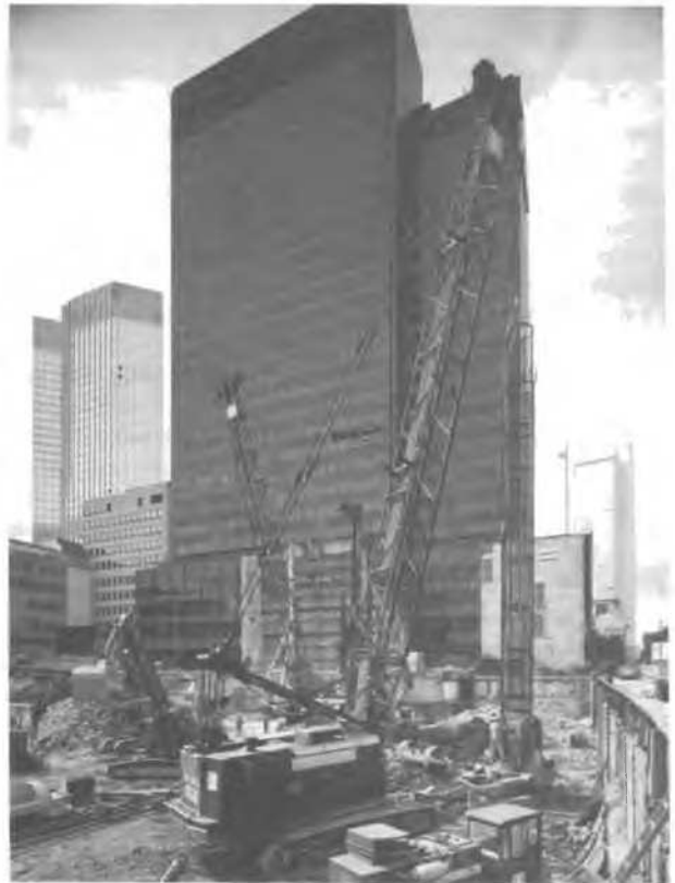
Figure 1 Pile installation for the new Commerzbank office in Frankfurt
