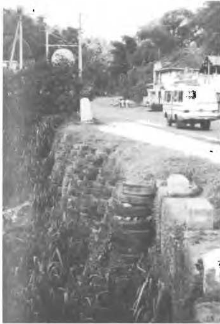
Plate 3 - Completed Anchored Tyre Structure at Ranwala
