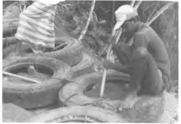
Plate 2 - Compaction of Fill Inside the Tube Space
