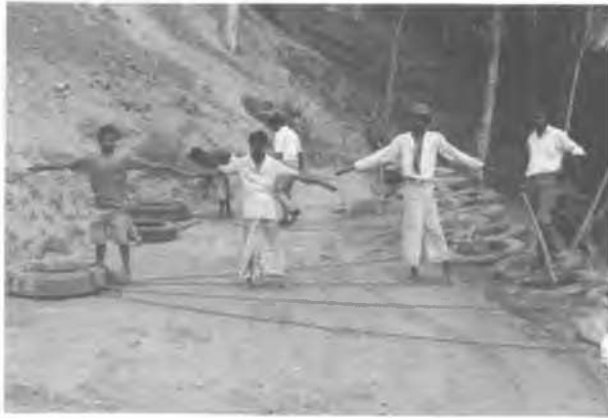
Plate 1 - Placement of Anchor and Facing tyres
