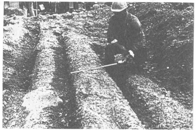
Fig. 3 Excavated Soilcrete trial field
