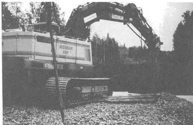
Figure 7. Block stabilization in Ranea in northern Sweden.
