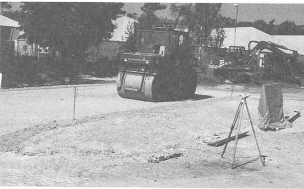
Figure 9. Compaction of the covering mineral layer
